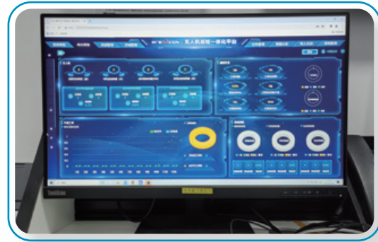
Autonomous UAV inspection platform
